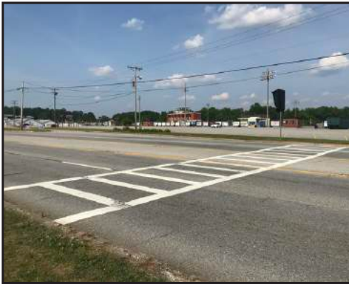
Unsignalized midblock crossing across 5 lanes of traffic (US-176); sidewalk gaps on both sides
